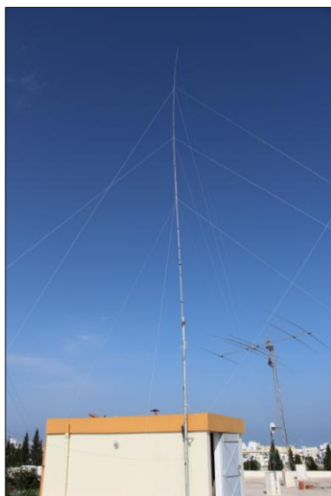
Figure 17: the new 80m Antenna in 3V8SS
